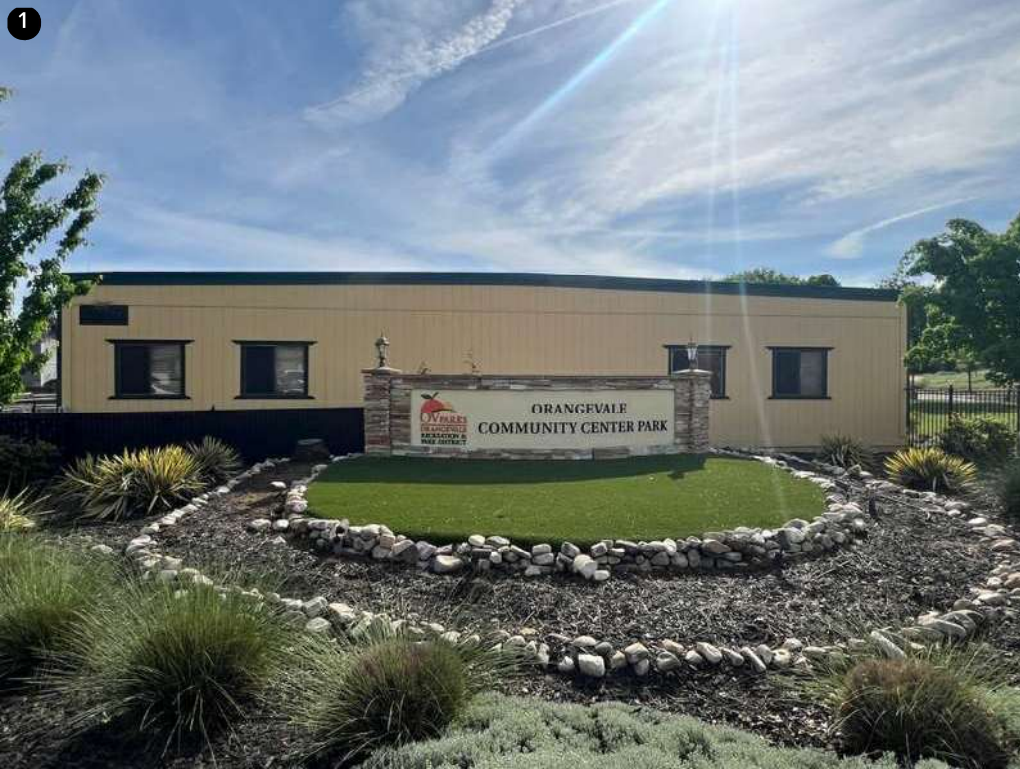
1 Overview. The perimeter edge metal, gutters and downspouts looks great!
