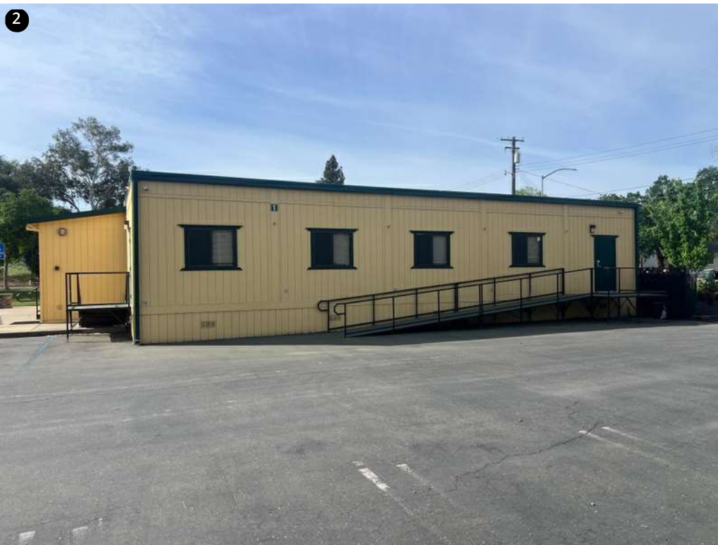
2 Downspouts installed and the entire work area clean.
