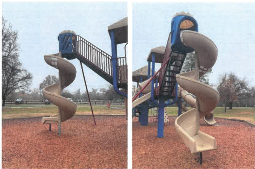
Large slide repair & replace at Orangevale Community Park
