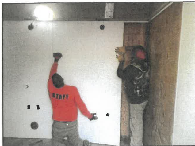
Pecan Park Restroom Repairs
