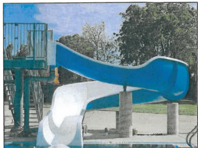
Pool Slide with New Paint and Gelcoat
