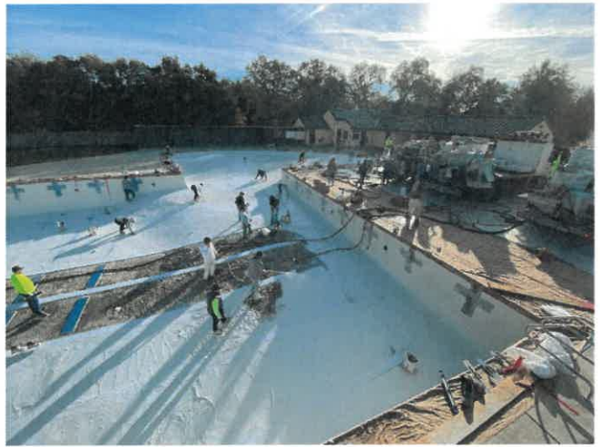
Apply plaster to the pool (12/5/23)
