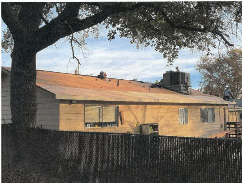
Back roof with new plywood sections (12/5/23)
