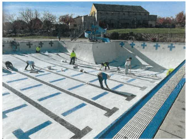
Smoothing the plaster and cleaning the tile (12/5/23)
