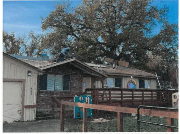
Replacing plywood on section of roof (12/5/23)
