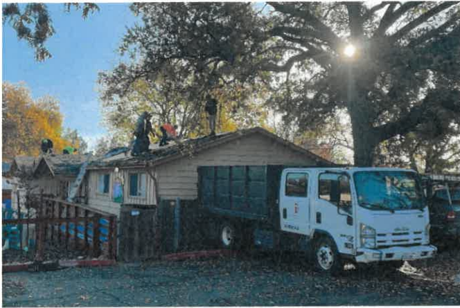
Removing old roof (12/4/23)
