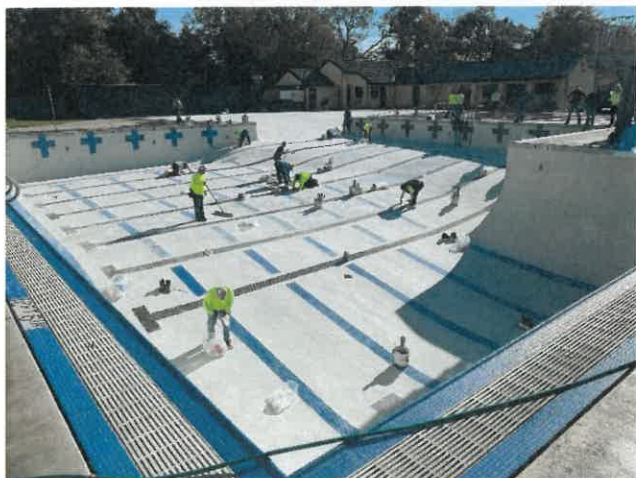
Smoothing the plaster and cleaning the tile (12/5/23)
