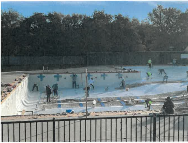
Apply plaster to the pool (12/5/23)
