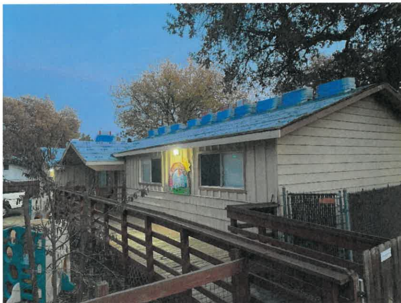
Roof is protected for upcoming rain (12/5/23)
