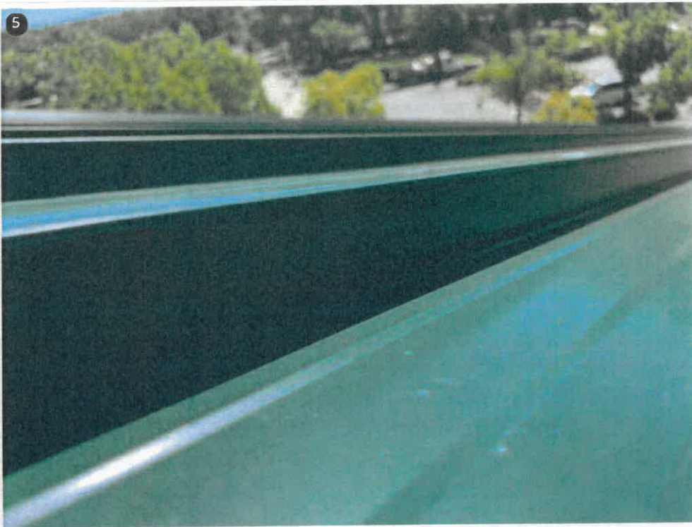
5 Upclose of the ridge cap installed and seamed.
