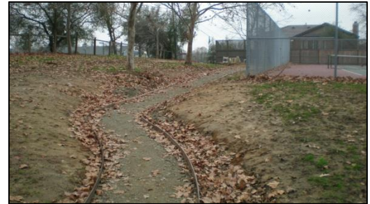
Figure 42 - New Sidewalk Under Construction Near Tennis Courts
