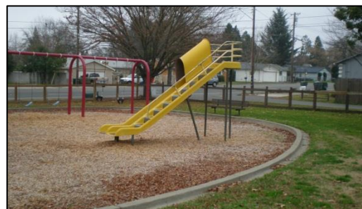
Figure 70 - Playground Area Safety Hazard Equipment
