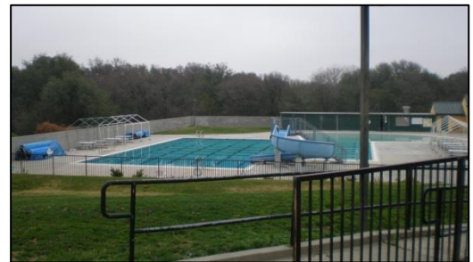
Figure 46 - Orangevale Community Center Pool
