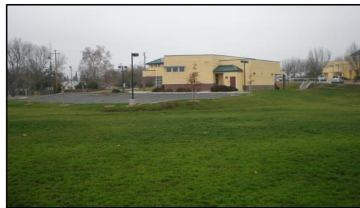
Figure 50 - Un-level Grading in Diamond Outfields
