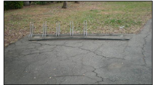
60 Figure 66 - Damage Bike Rack and Cracked Hard Surface Trail
